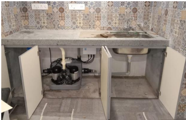
Sanicom 2 installed in the kitchen
