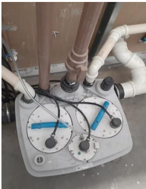
Sanicubic 1 WP installed in the basement
