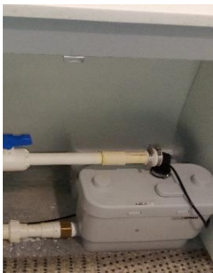
Sanispeed installed under the sink
