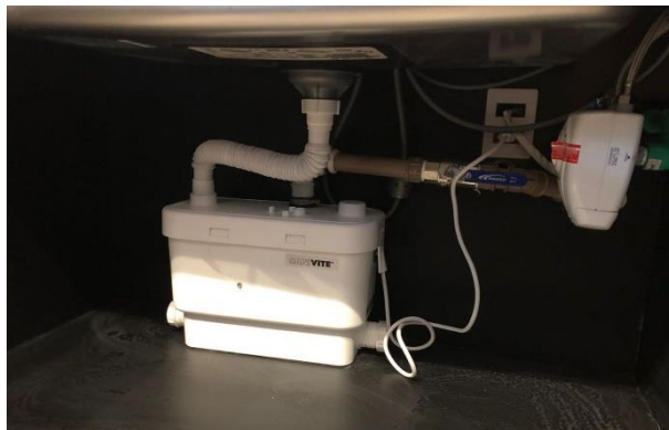
Sanivite installed under the kitchen sink in the basement bar
