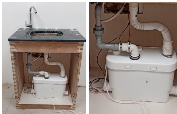
Sanivite installed in the office pantry
