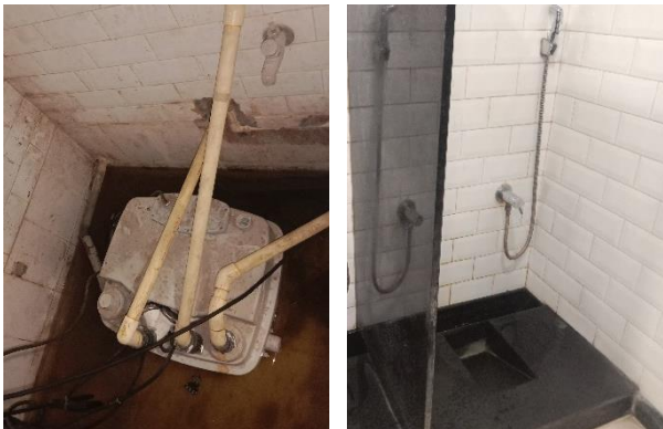
Sanicubic 2 Classic pump installed and connected
