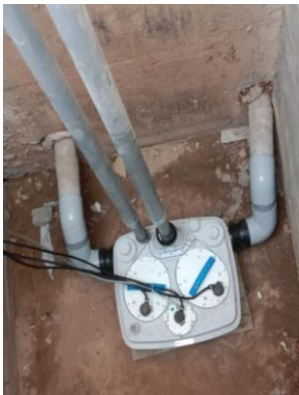
Sanicubic 2 Classic installed in the basement
