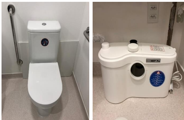
Sanibest Pro installed behind the toilet
