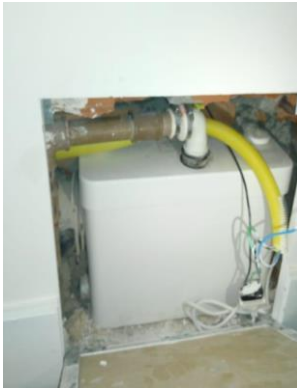
Sanipack installed behind the bathroom wall
