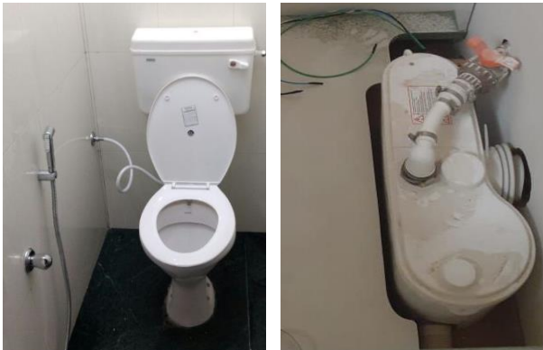
Sanibest Pro installed in the washroom behind the wall of the WC
