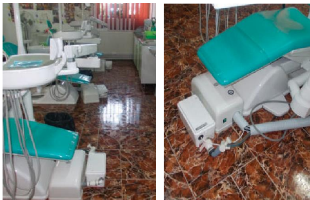
Sanishower pumps installed to drain wastewater from the sinks
