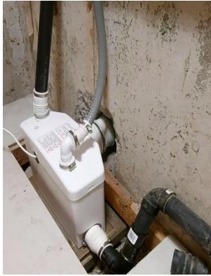
Saniaccess installed behind the washroom wall
