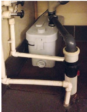
Sanispeed installed under the kitchen sink
