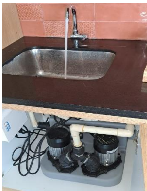
Sanicom 2 installed in the pantry
