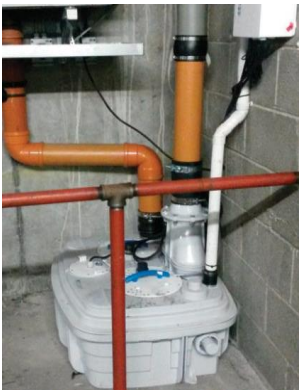
Sanicubic 2 VX installed in the equipment room
