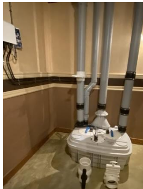
Sanicubic 2 VX installed in the basement
